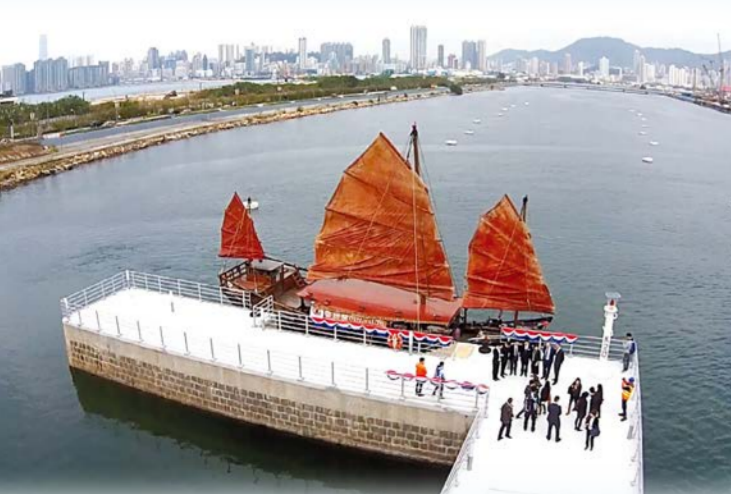
翻新後的跑道公園碼頭 Runway Park Pier after refurbishment works completed
