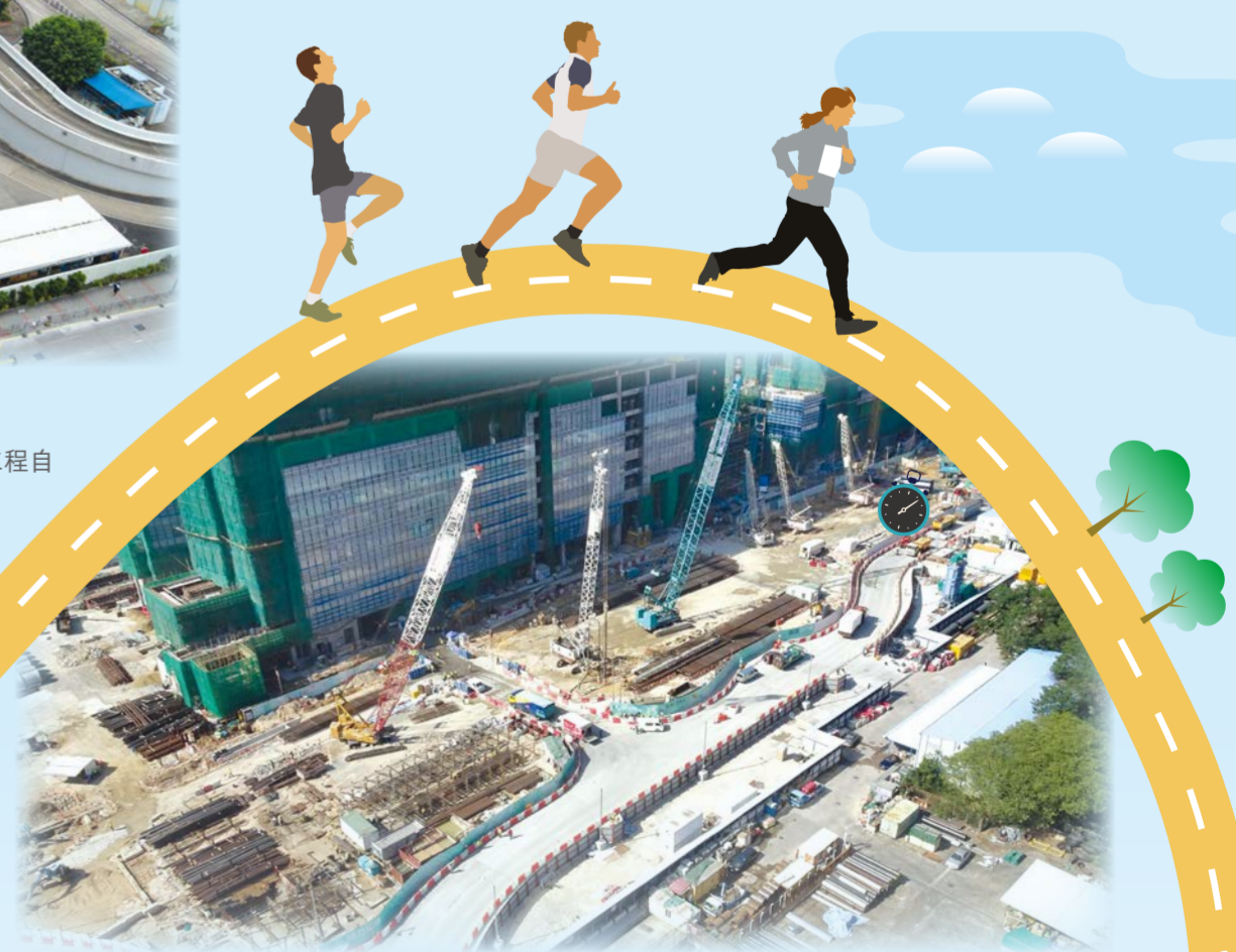
正進行的承昌道重建及地下結構興建工程 Reconstruction of Shing Cheong Road and construction of underground structures are in progress
