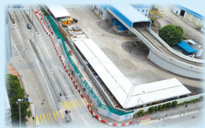
常怡道交匯處的道路擴闊工程 Sheung Yee Road junction widening works
